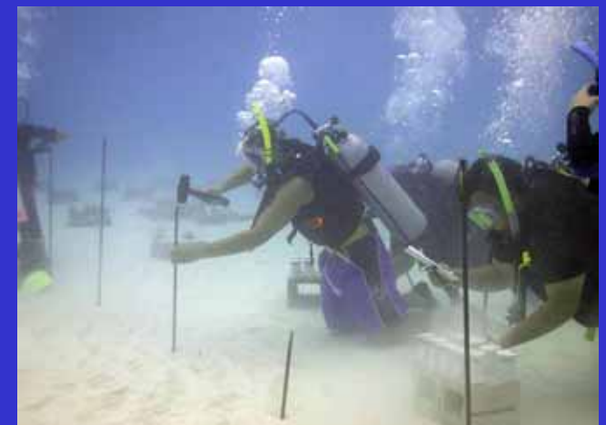
Pounding in rebar to anchor blocks
